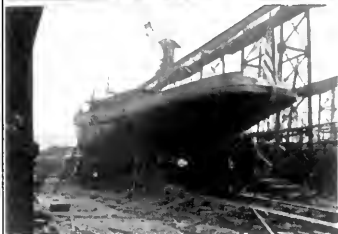
Above are three views taken at the launching of the twin-screw, steel towboat Mamor at the Potrero Works of the Bethlehem Shipbuilding Corp., Ltd., San Francisco, for Young Brothers of Honolulu. The vessel is 129.2 ft. long, powered by 750 H.P. Fairbanks-Morse Diesel engines.
